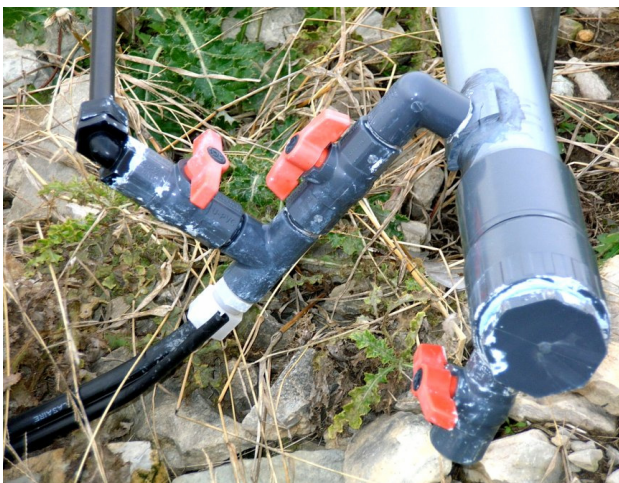
Typical High-Pressure Air Compressor Connection for Air & Drain Manifolds
