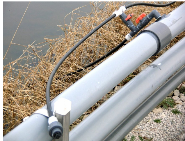
Moisture Purge Connection for Air & Drain Manifolds
